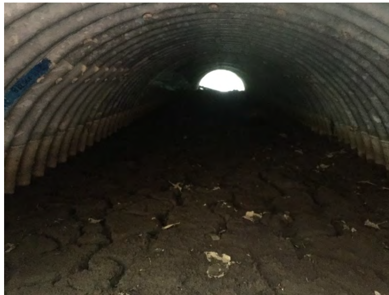
Looking through culvert from outlet
